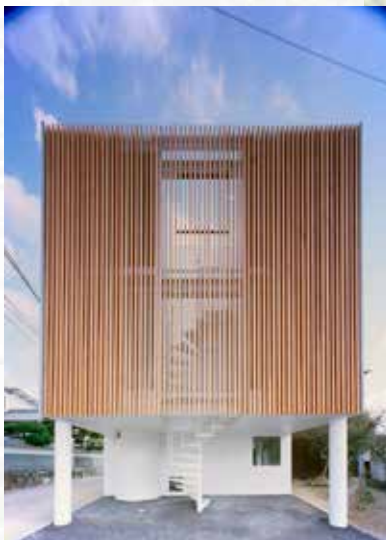
HK House Facade
